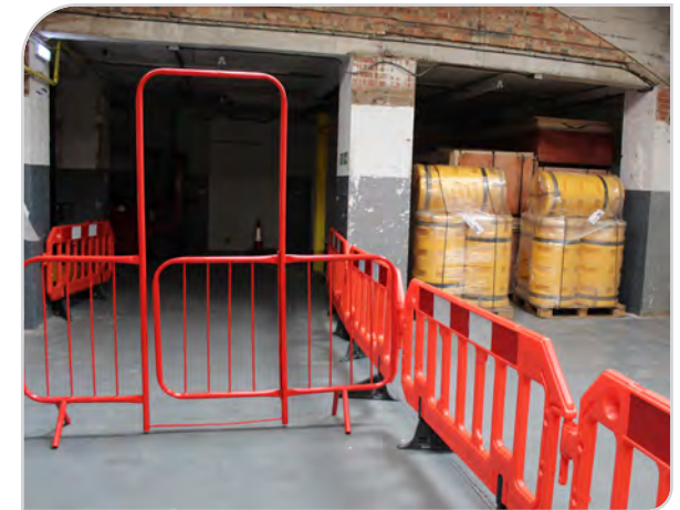
Walk through barrier at site in Worthing
